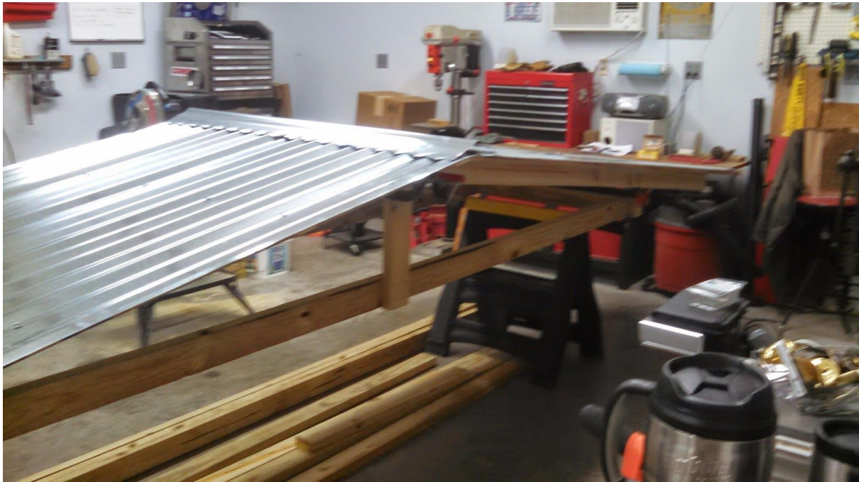
Photo showing an end pair of roof panels under construction. Note king post and truss bottom component.
