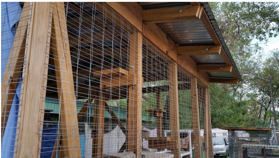
Photo showing roof overhang and connection details and platform attachment inside. Note that roofing tin extends past roofing stringers and rafters.
