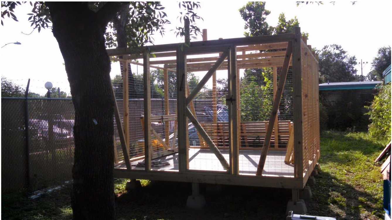
Photo showing all wall modules installed and bolted down. Note that roof section truss bottoms are in place along with king posts. Next step is to begin installation of roof panels starting at the far end.
