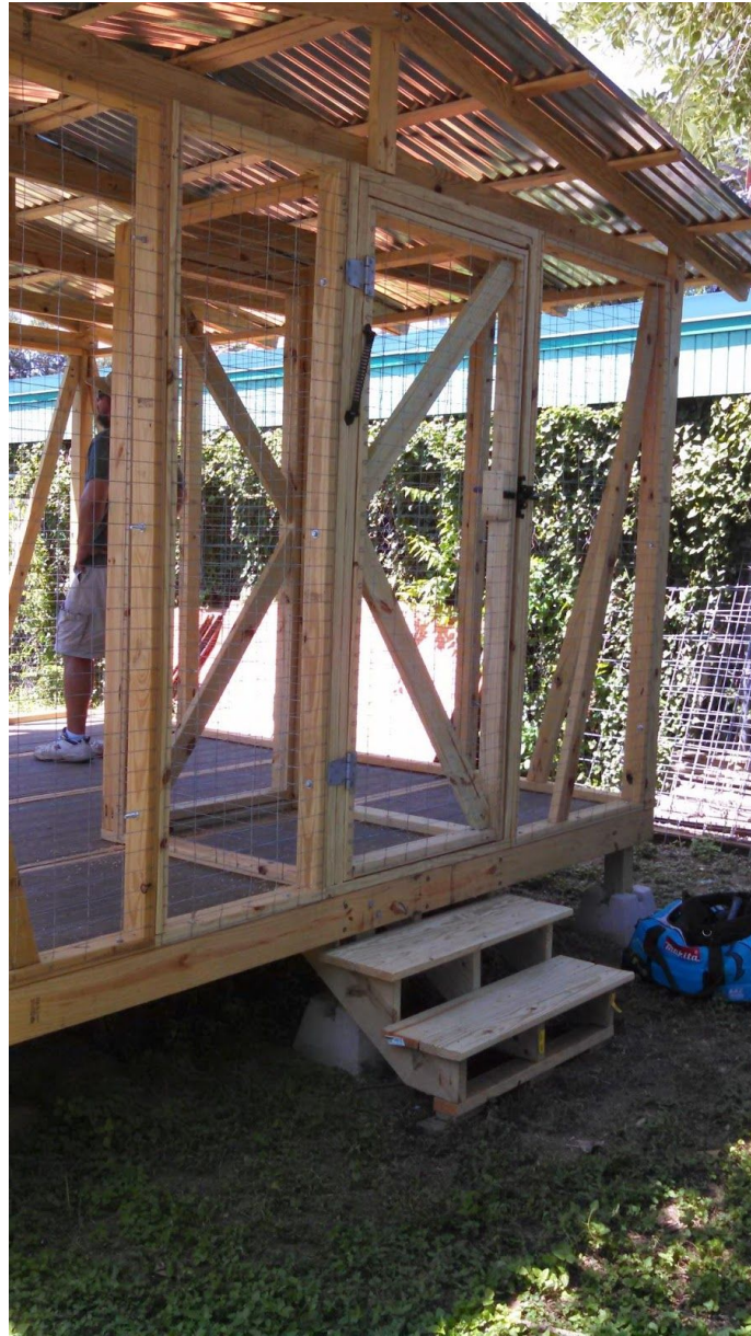
Photo showing modular sections, airlock and stairs.. Photo was taken before second layer of wire screening was added.
