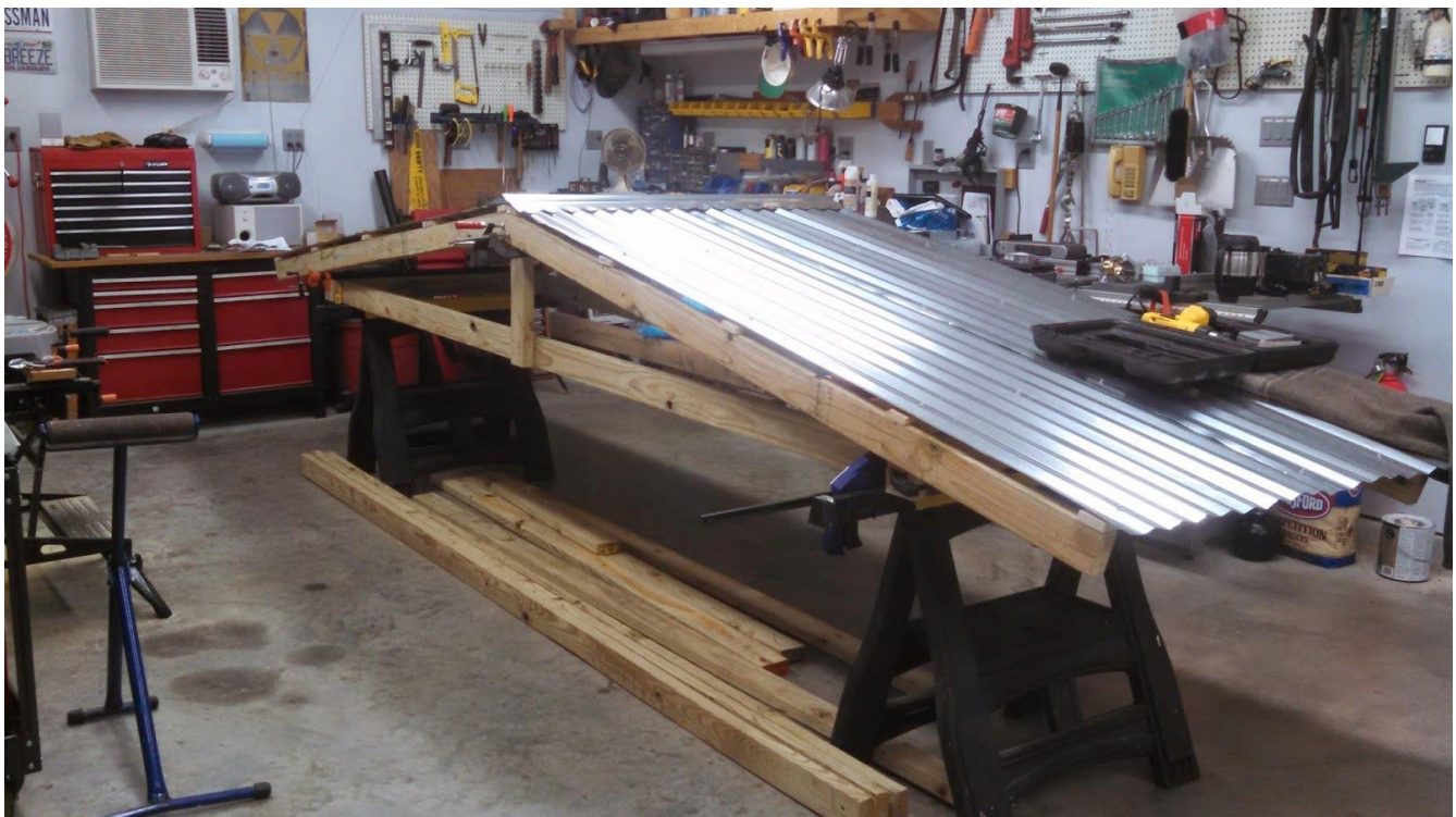
Photo showing back side of roof module pair (interior side) plus king post and truss bottom.
