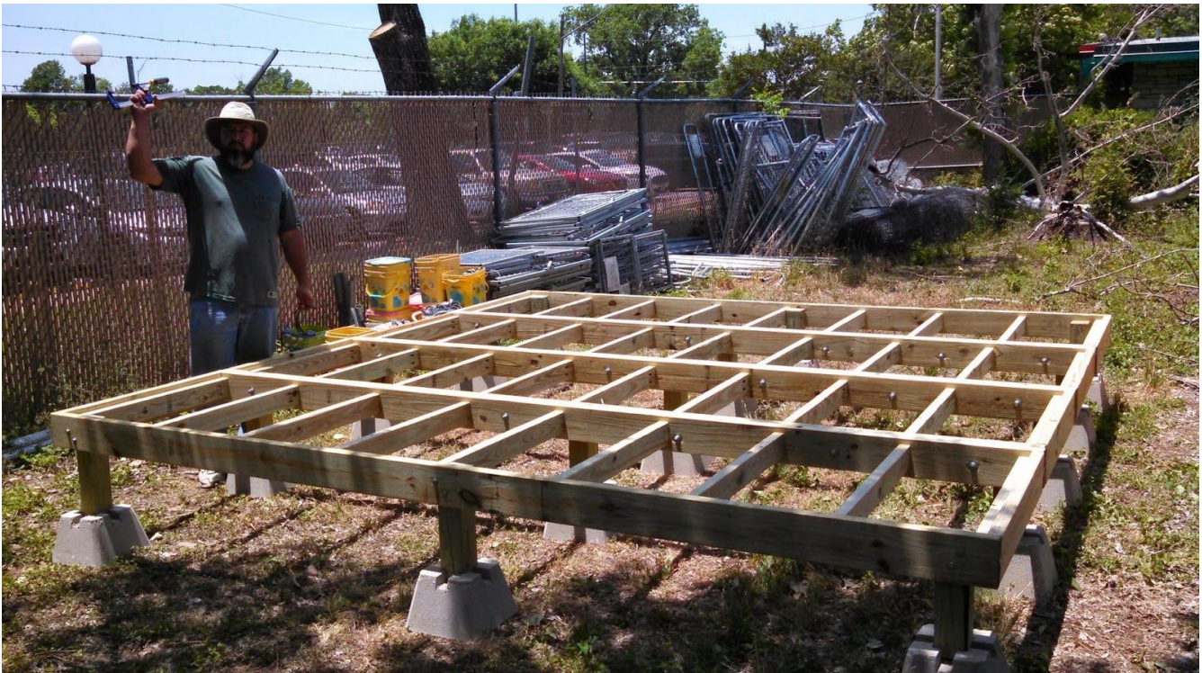
Photo showing all four modules bolted together with carriage bolts, footing posts and concrete anchor pads.
